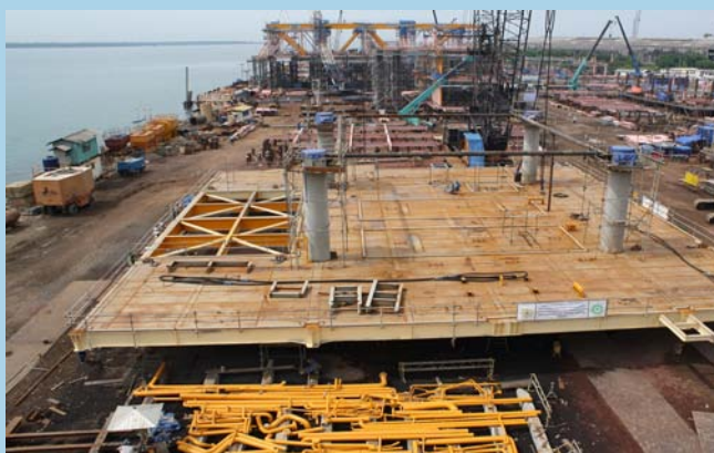
CPP Main Deck
